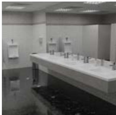
The Hands Free Faucet System operates entirely on water pressure using a pilot/slave valve pair instead of an electrical connection
