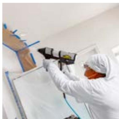
The texture sprayer and cartridge system makes the job of spraying texture on interior walls and ceilings faster, lighter, and more cost-effective
